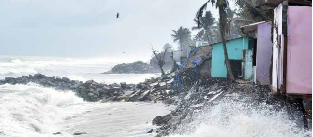
High swell waves hit the eroded shoreline of Anchuthengu, destroying houses, as a result of a storm in the Southern Ocean, 9000 km away from the Indian coast. (Photo: Kevin Julius)
